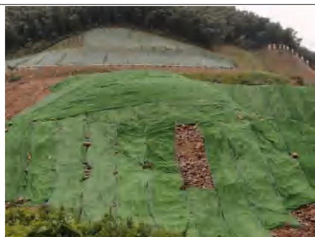
裸露边坡临时苫盖防护
