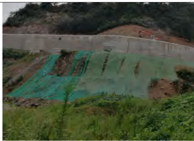
裸露边坡临时苫盖防护
