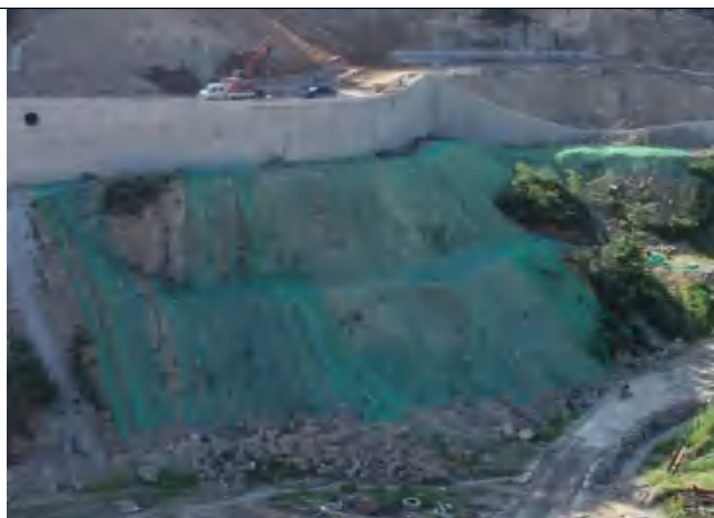
裸露边坡临时苫盖防护
