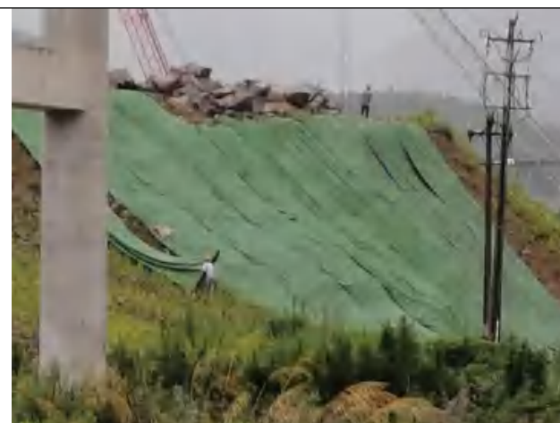
裸露边坡临时苫盖防护
